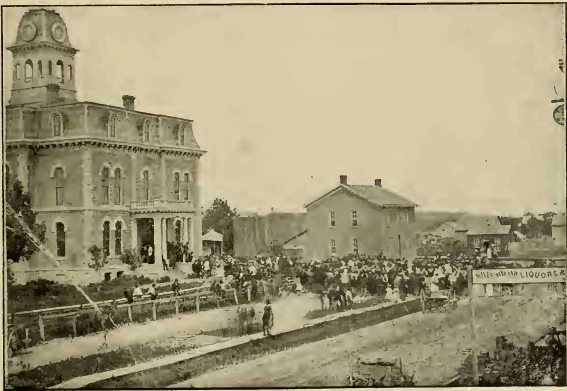
SCENE OF THE HANGING OF NATHAN BURGESS AT EFFINGHAM, ILL.
